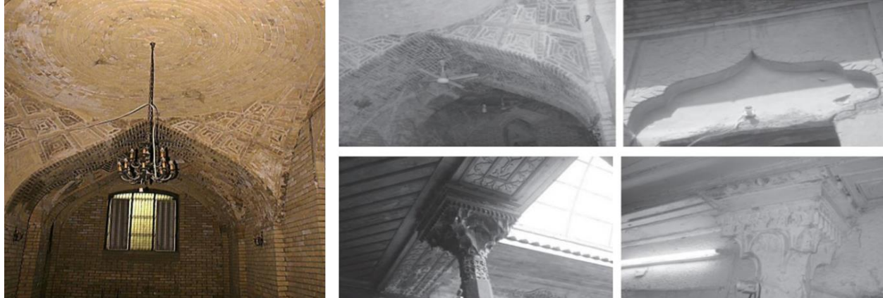
Figure 2. Decorative wooden columns along the edges, brick ceilings and arches, and Muqarnas ceilings [4].
