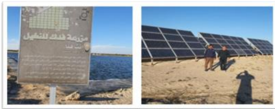
Figure 2. Fadk water pump project
