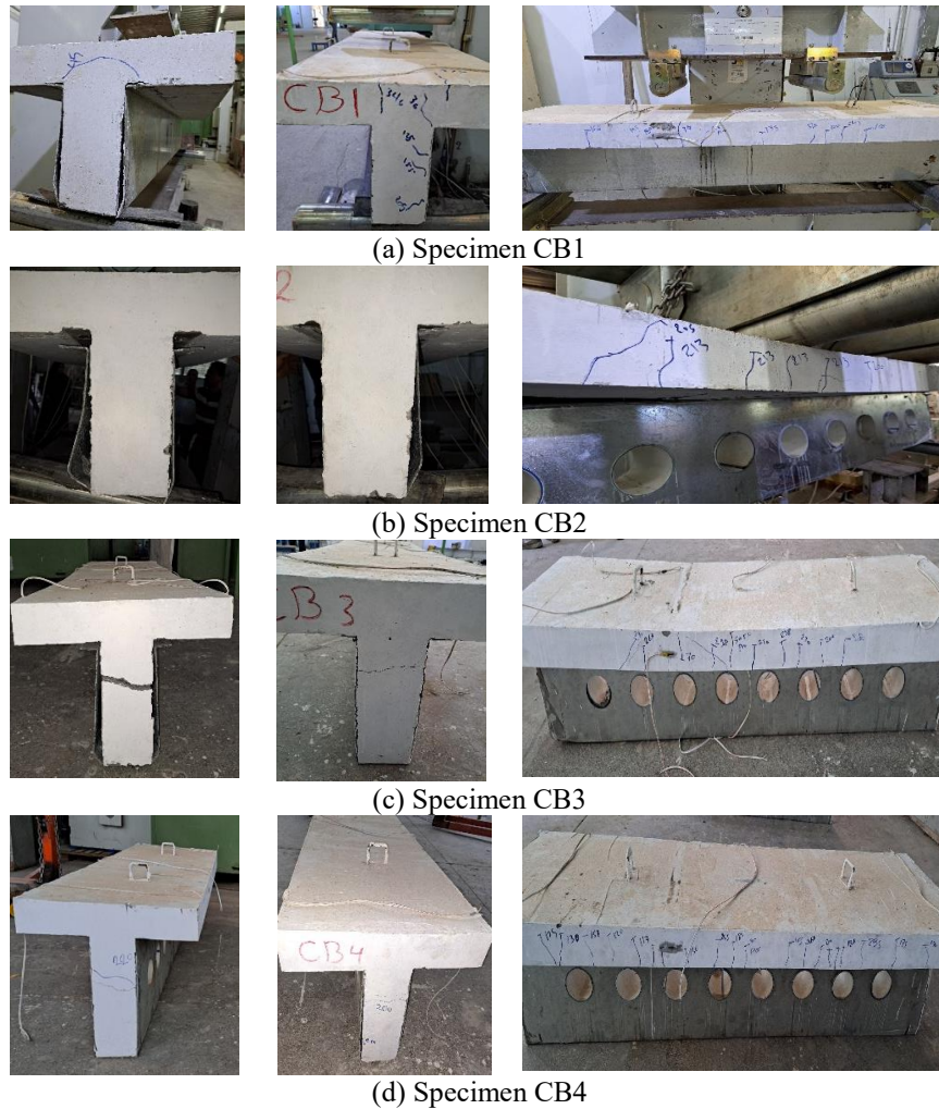
Figure 9. Composite beams after failure.
